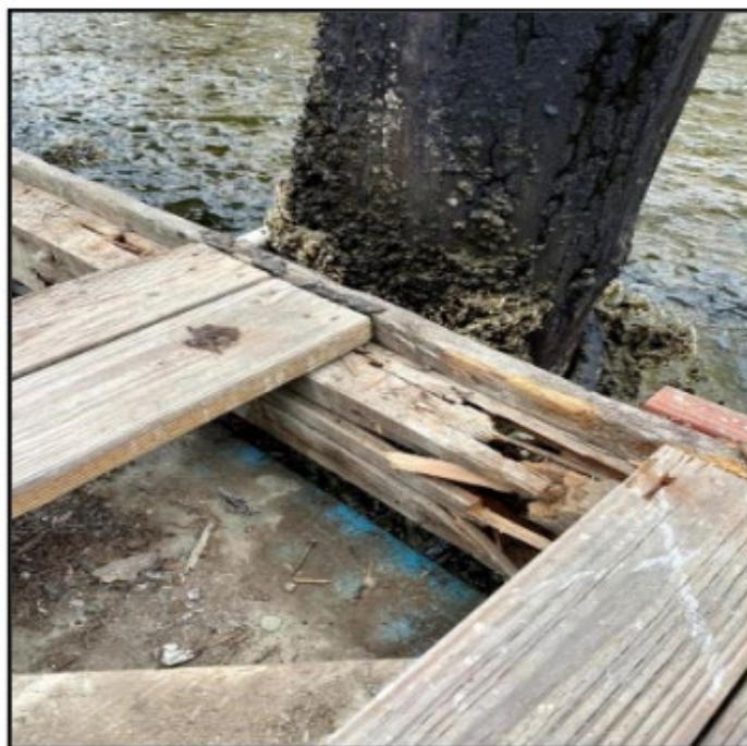
August 24, 2021 Site Inspection: Timber framing is broken at pile guide connection at East dock Pile 2
